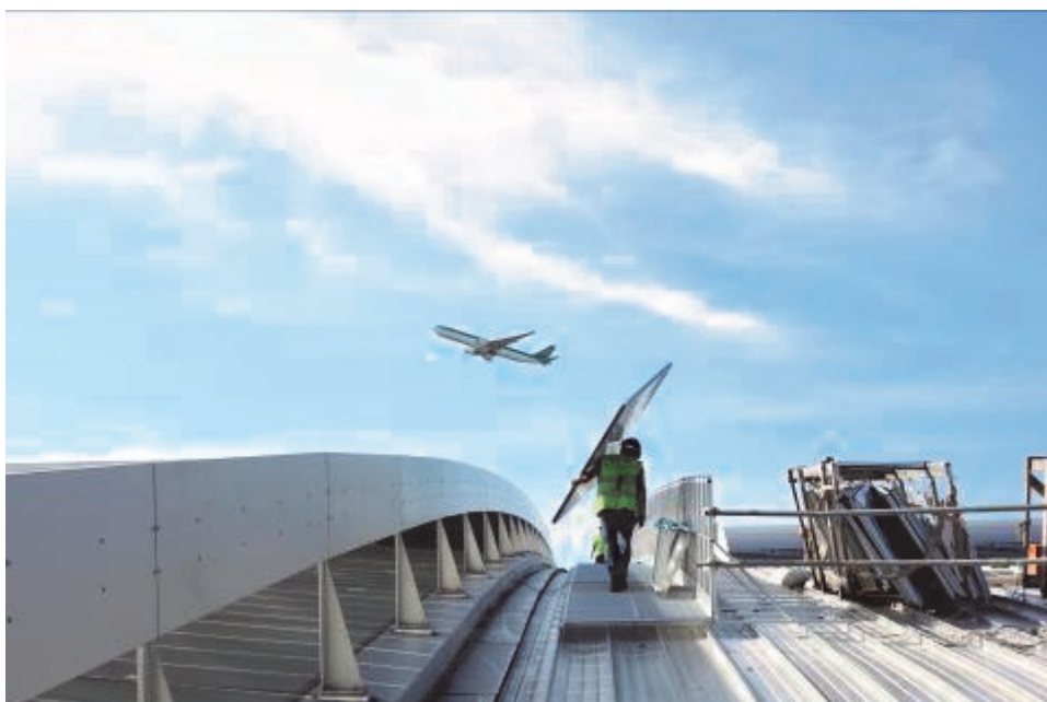
View of a construction worker carrying an external cladding panel across the roof of the new Terminal. The cladding and glazing contract for T2 is being delivered by the Portuguese firm, Martifer.
